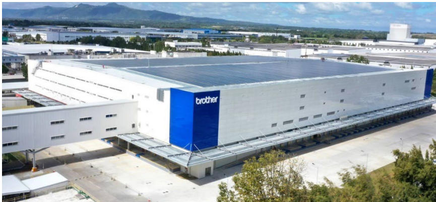
New factory building of Brother Industries (Philippines) (Factory No. 3)
